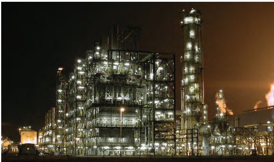
RUWAIS WorleyParsons will serve as project manager for the fourth phase of the massive petrochemical complex owned by Borouge.
